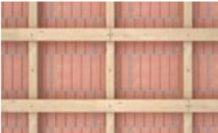
Timber façade substructures
